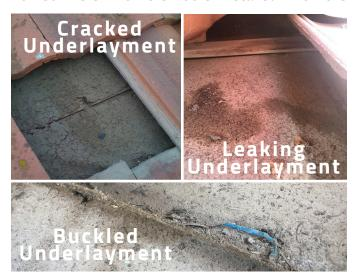
minimum required underlayment (30# felt) can expect 16-18 years of life. Having your paper inspected properly requires careful lifting and replacement of shingles or tiles in trouble areas. To avoid damage or incorrect re-fitting, it's best to consult a professional roofer for this type of inspection.
