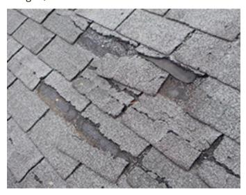
should also look for moisture stains on the underside of eves and overhangs. Scan for loose material or wear around chimneys, vents, pipes, or other penetrations. Also, make sure to look for cracked and worn mortar joints on tile roofs. If you have an older shingle roof, look for an excessive amount of shingle granules in the gutters or on the ground at the perimeter of your home.
