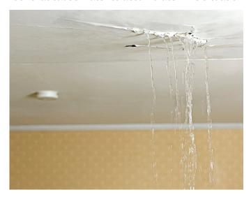
allows water to deteriorate the underlayment over time, and can eventually cause significant interior water damage. This can result from something as miniscule as a tear in the underlayment, or a crooked nail. The point is that roof leaks are not always sudden or storm related damage.
